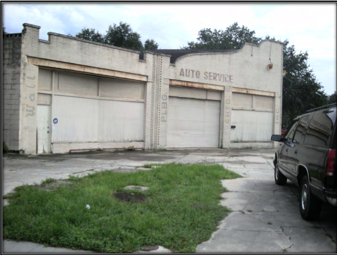
15. View facing south of the vacant auto service facility in the southwest section of the subject property.
