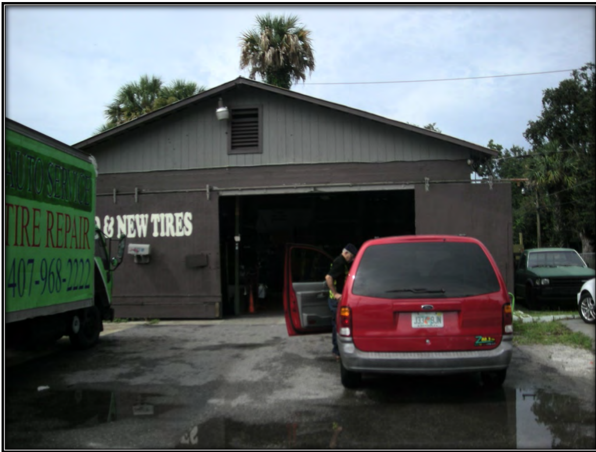
11. View facing south of the tire facility in the southwest section of the subject property.
