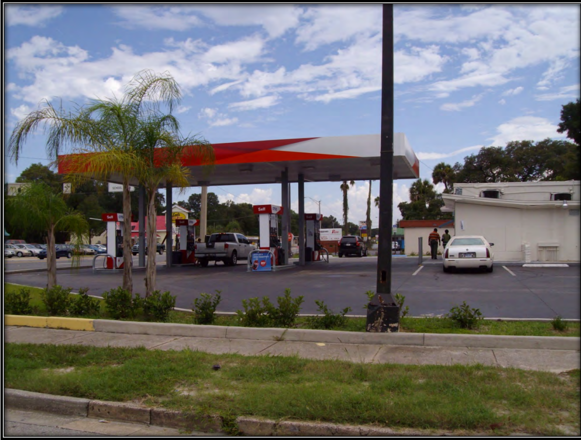
11. View of a gasoline station on the east side of the subject property, facing south.
