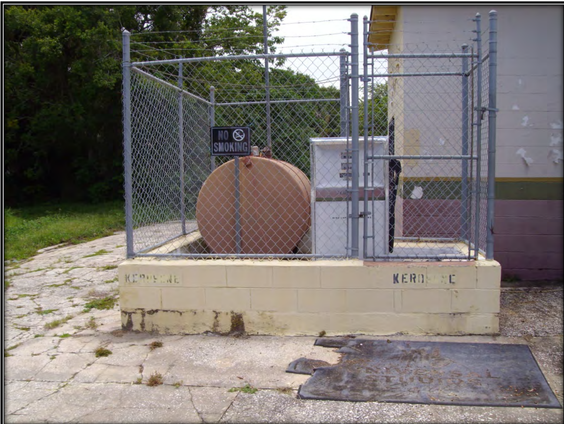
4. View of an approximately 500-gallon capacity kerosene AST behind a vacant business at 927 W. 13 th St.
