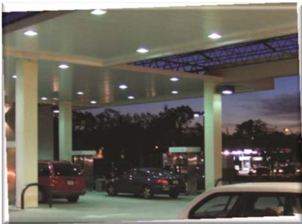
Recessed lighting creates a well-lit space without causing glare.
