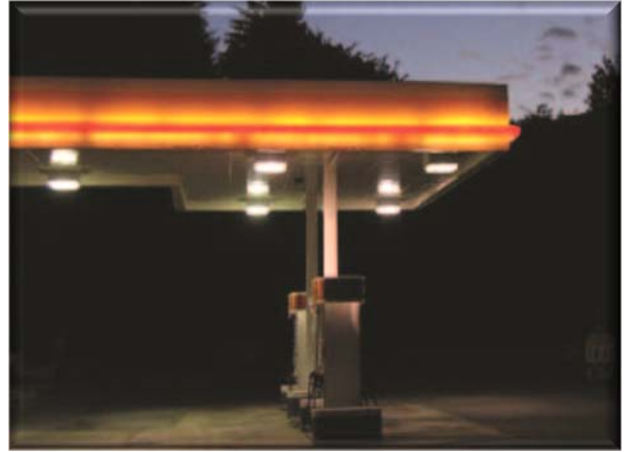
Lighting shall not be mounted on the sides of canopies. It causes unnecessary light pollution. Under canopy lighting shall be recessed.
