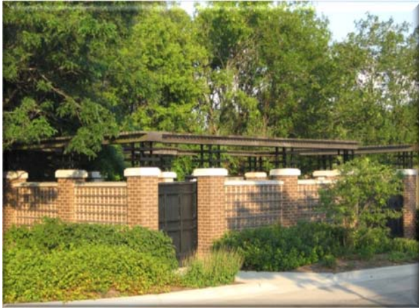
Dumpsters and utilities are suitably screened in a parking lot with an architectural wall, solid metal gate and a mixture of landscaping materials.
