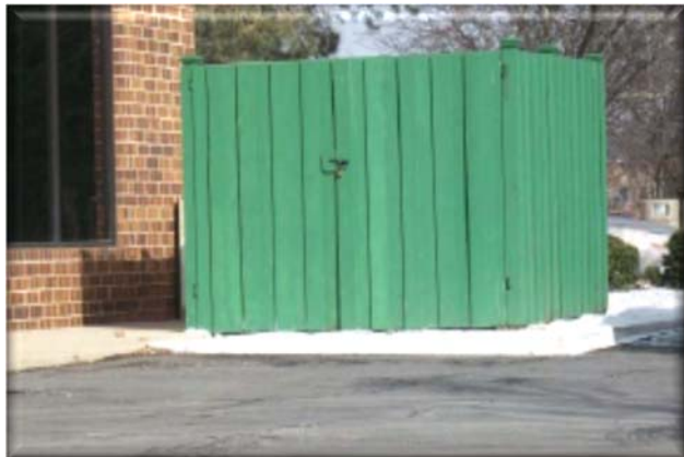
Screening materials should be compatible with the building architecture, rather than draw pedestrians' attention to the screen.
