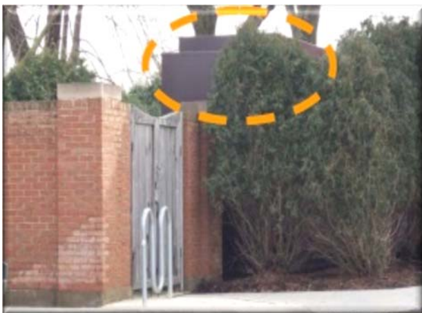
Brick piers, evergreen screening and a decorative wood gate screen a large generator.
