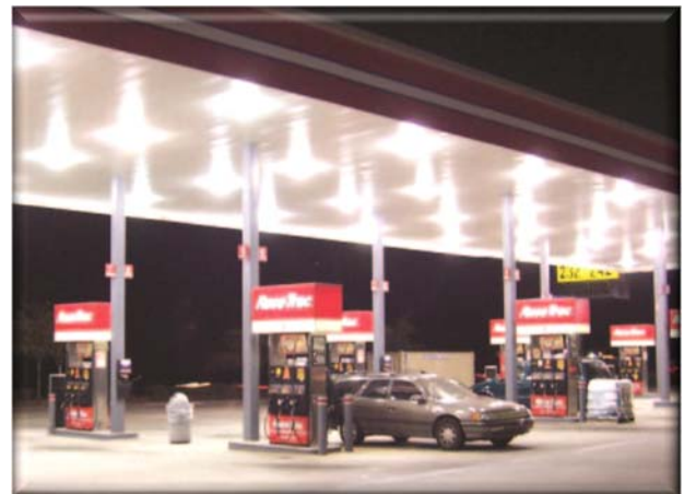
Globe fixtures result in glare and light pollution, as they emit light in all direction and are not recessed.
